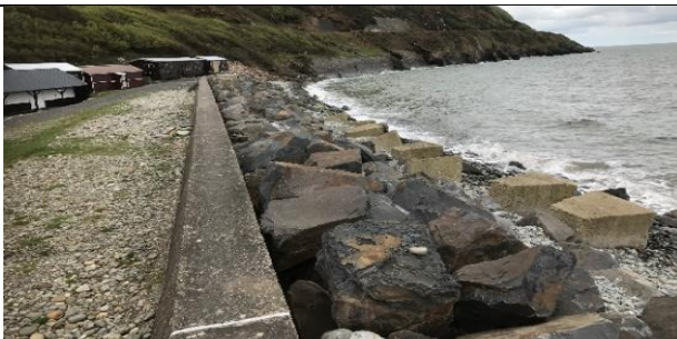
Figure 5. Protection measures and beach profile near Friog Cliffs at the southern end of Fairbourne Village
